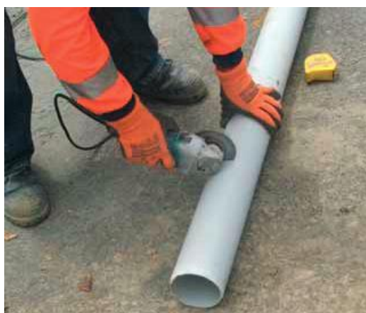
Figure 5 - Cutting pipe with power-driven masonry blade
