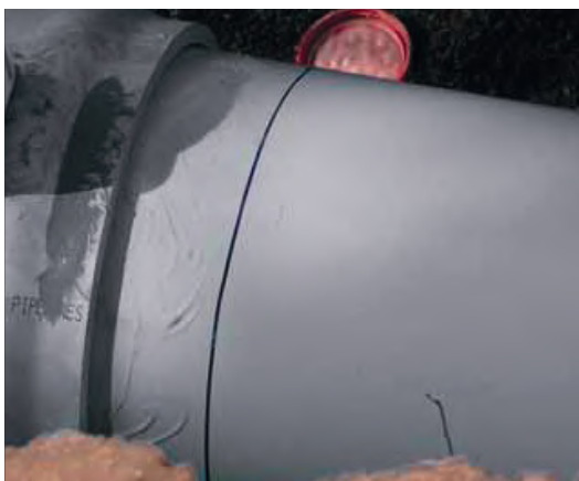
Figure 13 - Insert aligned lubricated spigot into socket
