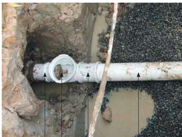
Figure 36 Typical positioning of hydrostatic test plug
