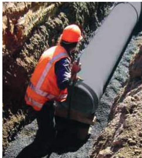
Figure 18 - Push joint home until witness mark remains just visible
