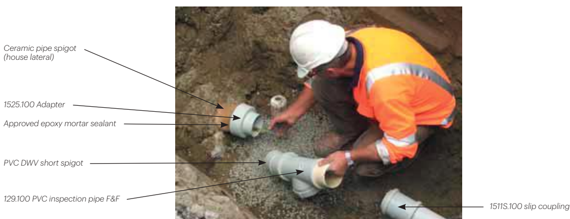
Figure 34 Ceramic Socket to PVC Adapter typical installation
