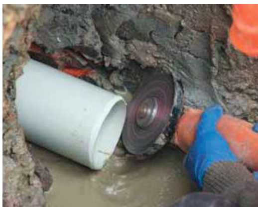
Figure 7 - Chamfering pipe with power-driven masonry blade
