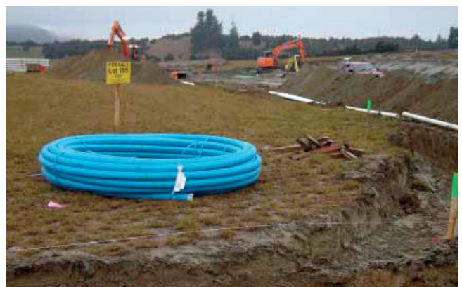
Coil of DN 63 PN 12.5 Iplex BlueLine polyethylene pipe on site, near Lake Wanaka.
