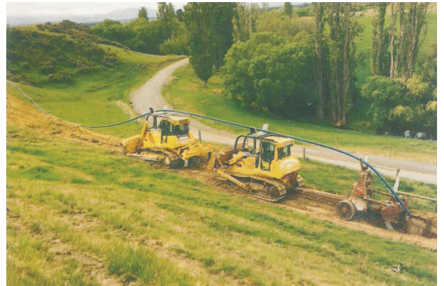
Mole Plough installation of Iplex Blackline pipes.
