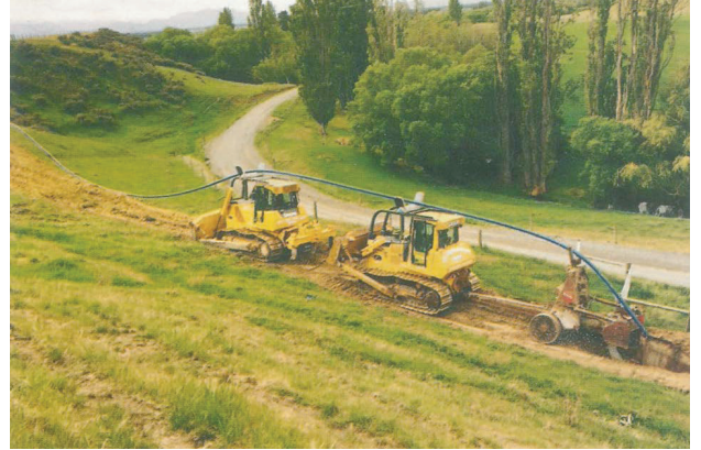
Mole Plough installation of Iplex Blackline pipes.
