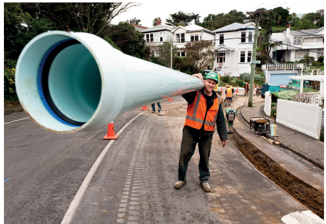
Manual site handling of light weight DN 150 S2 PN 16 APOLLO™ BLUE.
