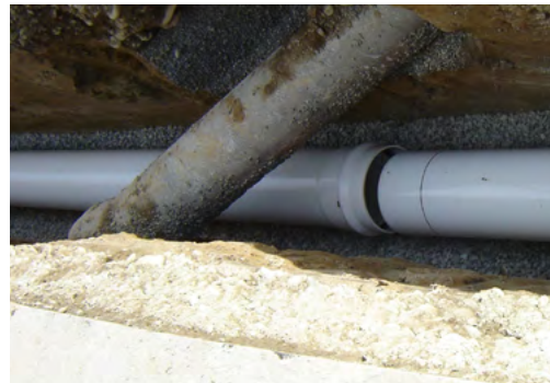
Figure 7.17 - Align the lubricated spigot with the socket mouth
