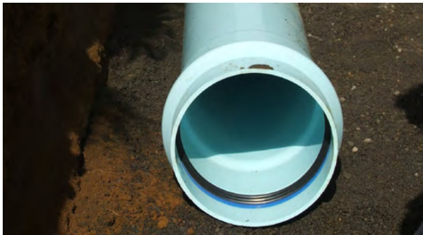
Figure 7.11 - Totally clean socket, ready for jointing
