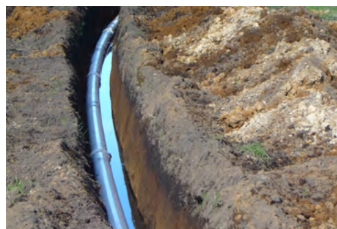
Figure 7.29 - DN150 Iplex Apollo® PVC-O Series 1 PN10 watermain, in 6m lengths, on a curved alignment, Hawkes Bay District
