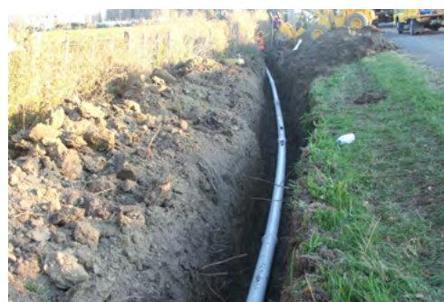
Figure 7.30 - DN100 Iplex Apollo® PVC-O Series 1 PN12.5 waste water transmission main, in 6m lengths, on a curved alignment, Gisborne District
