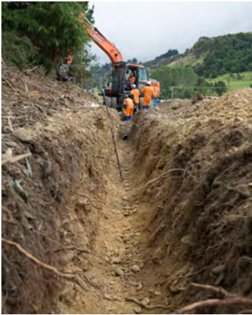
Figure 7.24 - Trench bottom in stoney ground, evenly cut to grade and depth before placing the bedding aggregate. Waitaki District
