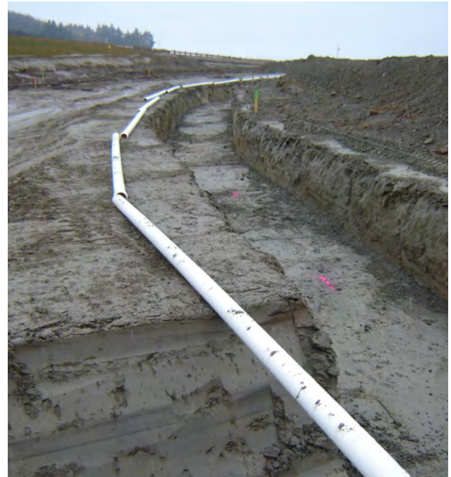
Figure 5.11 - Installing DN100 S1 PN12.5 Iplex Apollo® PVC-O pipes in sub-zero winter conditions, for a reticulation Water Main, Wanaka, Queenstown Lakes District
