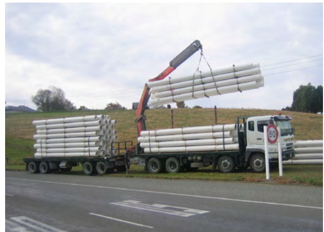
Figure 7.2 - Mechanical lifting, using two point suspension, and polymer slings, of DN300 Series 1 PN12.5 Iplex Apollo® PVC-O pipe in bulk crates, Timaru City
