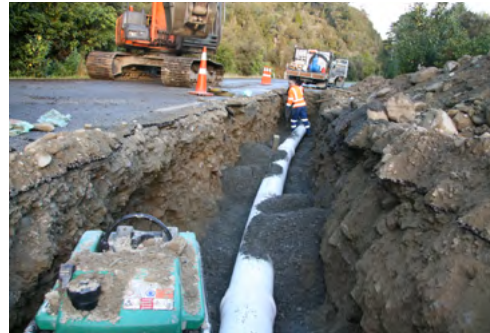
Figure 7.27 - DN300 Iplex Apollo® PVC-O Series 1 PN12.5 watermain in 6m lengths, following a curved road alignment, Westland District
