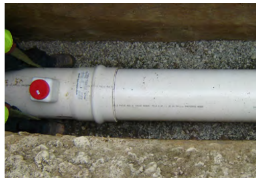
Figure 7.21 - Push joint home until witness mark remains just visible
