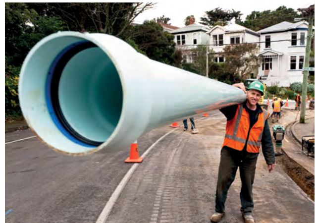
Iplex Apollo® Blue PVC-O DN150 PN16 pressure watermain, installed in Kelburn Parade, Wellington City, in 2011, specifically to improve seismic resilience in the area, which endured the November 2016 Kaikoura/ Culverden Earthquake sequence, undamaged.
