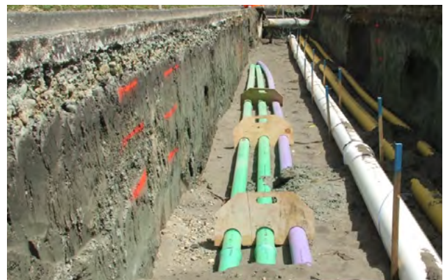
Figure 6.2 - Trench with temporary red index marks on the trench wall to guide backfilling and compaction in 300mm layers
