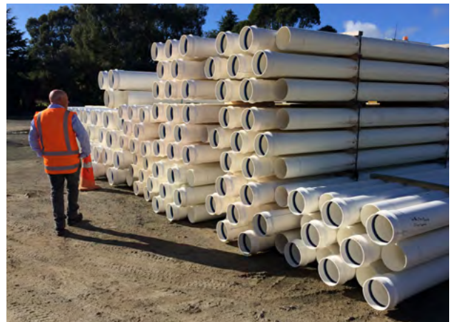
Figure 7.3 - Temporary storage of DN150 Series 1 Iplex Apollo® PVC-O pipe, in original factory crates on a flat site, near Oamaru, Waitaki District
