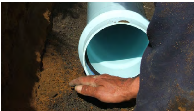
Figure 7.10 - Carefully clear away any dirt from the socket mouth
