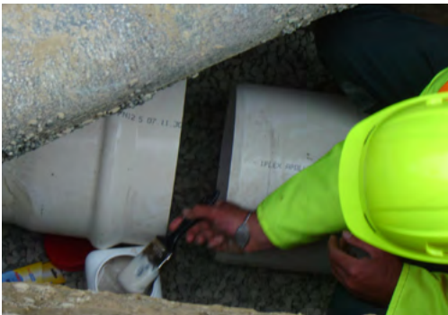
Figure 7.16 - Apply Medlube lubricant to both the seal and the spigot with a clean brush
