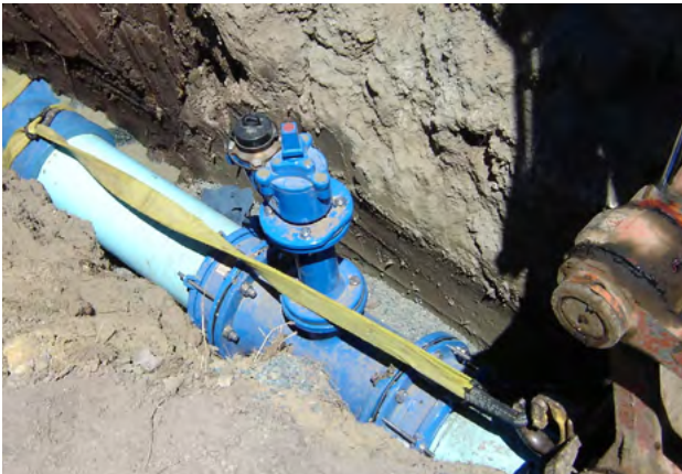
Figure 4.7 - Larger size ductile iron fittings may need extra mechanical help to assemble, such as here, with a lifting strop pulled by the excavator. DN250 socketed bend being assembled onto a DN250 Series 2 PN16 Iplex® PVC watermain near Richmond, Tasman District
