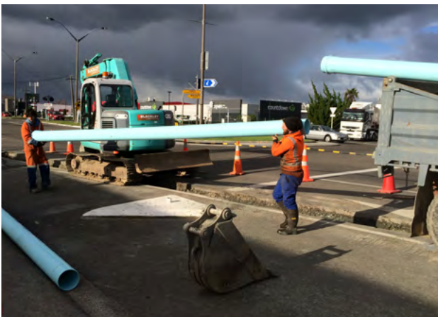
Figure 7.1 - Handling and unloading of DN150 PN12.5 Iplex Apollo® PVC-O pipe, preventing abrasion damage from the truck deck or by impacting the road surface. - Feilding, Manawatu District
