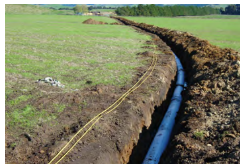
Figure 7.28 - DN300 Iplex Apollo® PVC-O Series 1 PN10 watermain in 6m lengths, on a curved alignment, Hawkes Bay District
