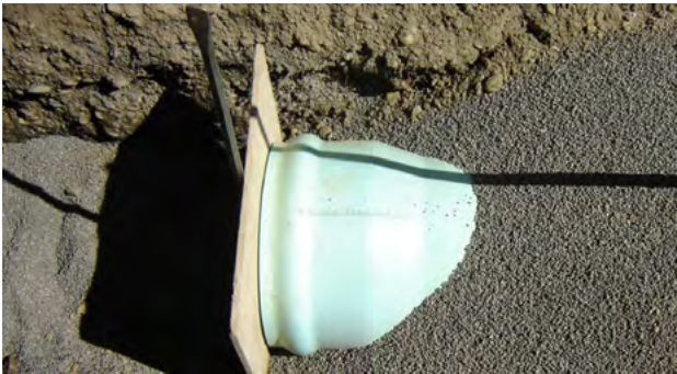
Figure 7.12 - Protect the clean socket from entry of dirt and grit, before joint assembly
