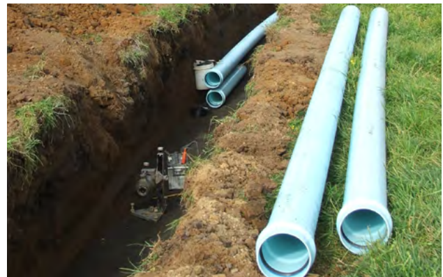
Figure 5.7 - DN150 S2 PN16 Iplex Apollo® PVC-O pipe used for a pressure sewer rising main - New Plymouth City, Taranaki
