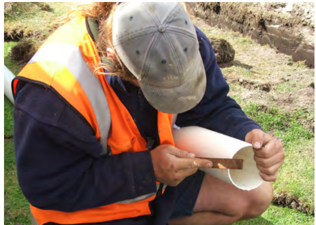
Figure 7.8 - Chamfering pipe with hand file
