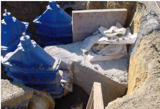
Figure 6.4 - Concrete thrust block supporting a three-way valve assembly, on a PVC transmission water main, Timaru City
