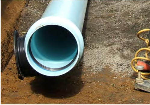
Figure 7.14 - Thoroughly clean seal ring and socket interior. Clear a small space under the socket to ensure the lubricated spigot does not touch the trench or pick up any dirt
