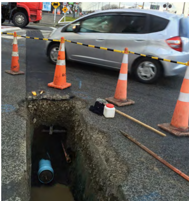
Figure 6.1 - Iplex Apollo® PVC-O, DN150 S2 PN12.5 installed under SH 54, Feilding Town Centre, Manawatu District
