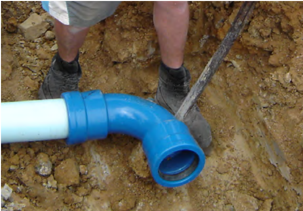
Figure 4.6 - Assemble the fitting onto the PVC pipe with a bar. Insert the pipe into the full length of the fitting socket
