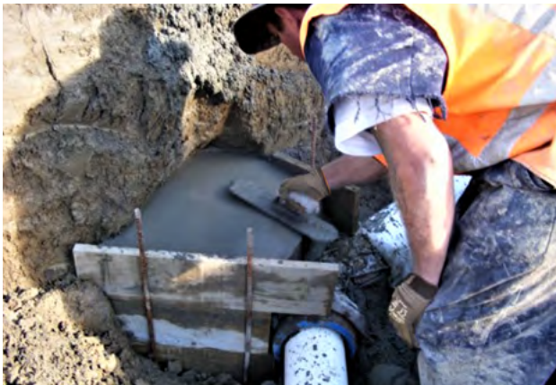
Figure 6.5 - Installing a concrete thrust block on a DN100, 45 Deg Ductile iron bend, fitted to Iplex Apollo® PVC-O PN12.5 pipe, Southland District
