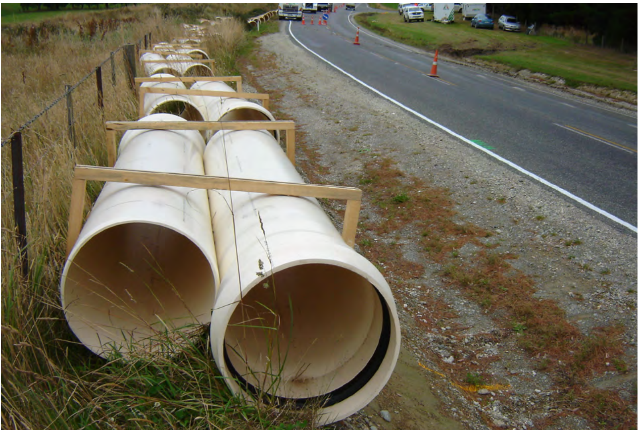
Iplex White Rhino® Series 1 PVC-M pressure pipe, used for a wastewater bulk transmission main.
