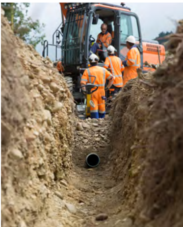
Figure 7.26 - Showing correct position of pipe, fully surrounded by selected size imported bedding aggregate, with all other larger size "as dug" aggregate, totally excluded from direct contact with the pipe, Waitaki District
