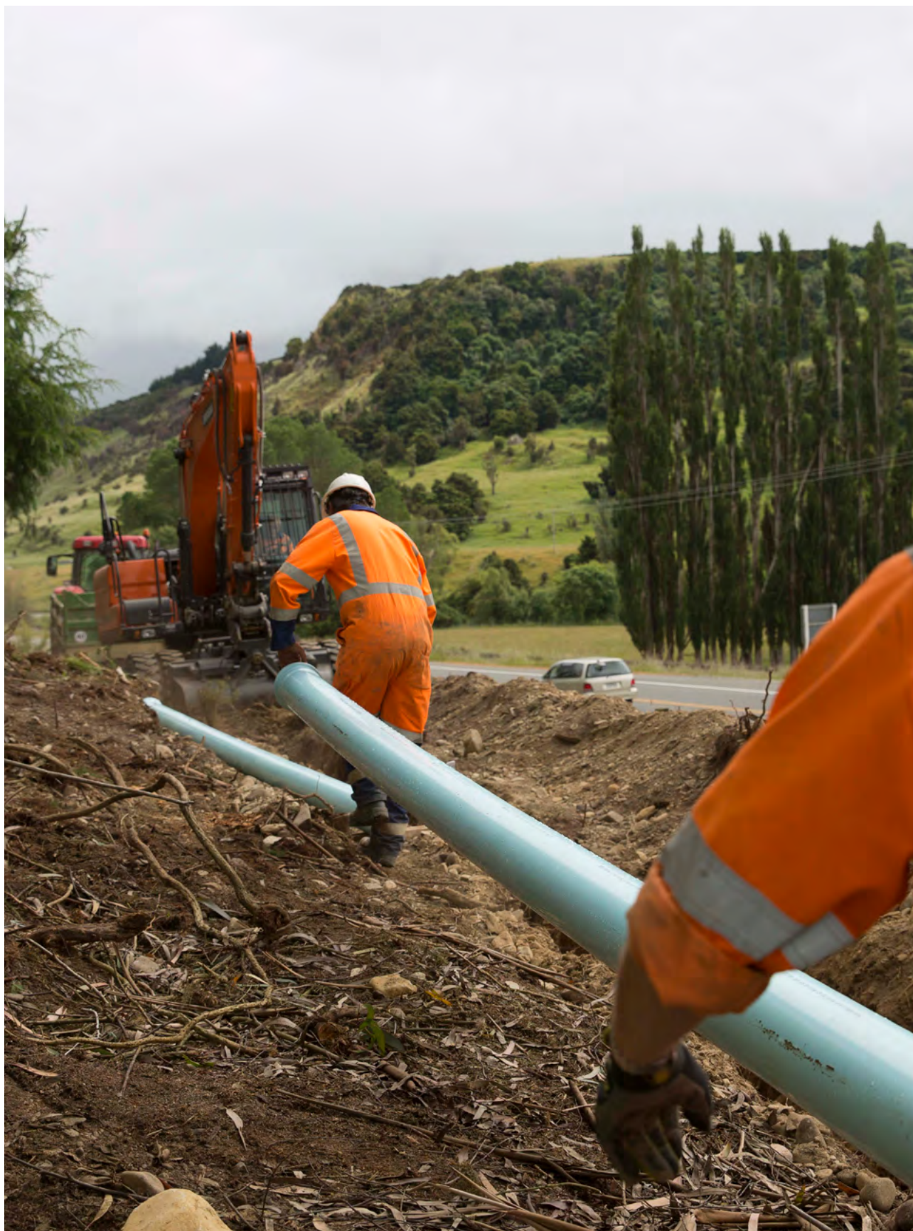
Iplex Apollo® Blue PVC-O Series 2 pressure pipe used on the Oamaru to Hampden Pipeline, Waitaki District.
