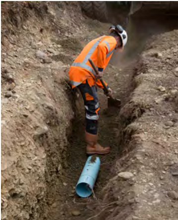
Figure 7.25 - Placing the selected size imported bedding aggregate, fully surrounding the pipe, Waitaki District
