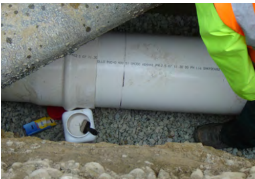
Figure 7.18 - Insert aligned lubricated spigot into socket
