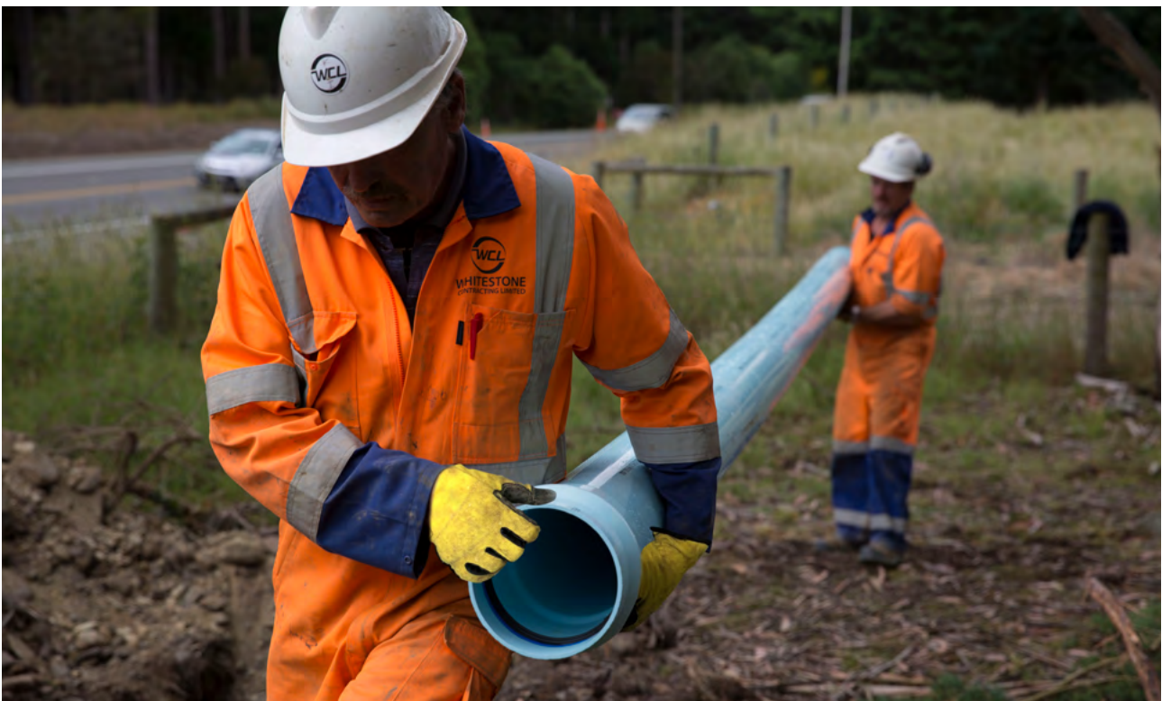
Iplex Apollo® Blue PVC-O Series 1 pressure pipe used on the Oamaru to Hampden Pipeline, Waitaki District.
