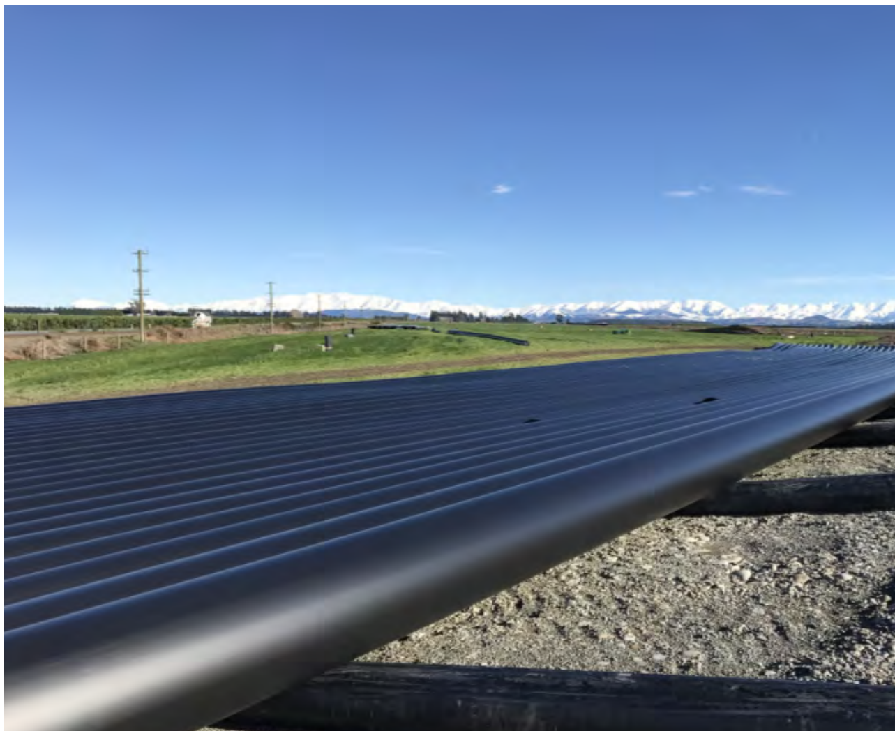
Iplex® PE 100 pressure pipe extruded on site in the Central Plains, Canterbury District.
