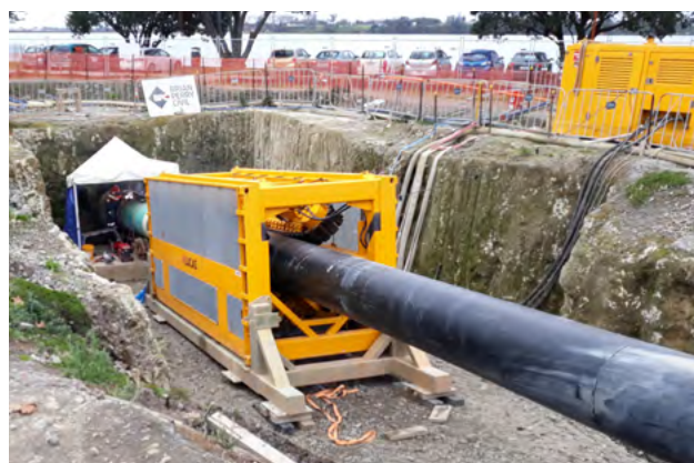
Iplex Poliplex® PE 100 pressure sewer transmission main, installed by Slip Lining, Tauranga City.
