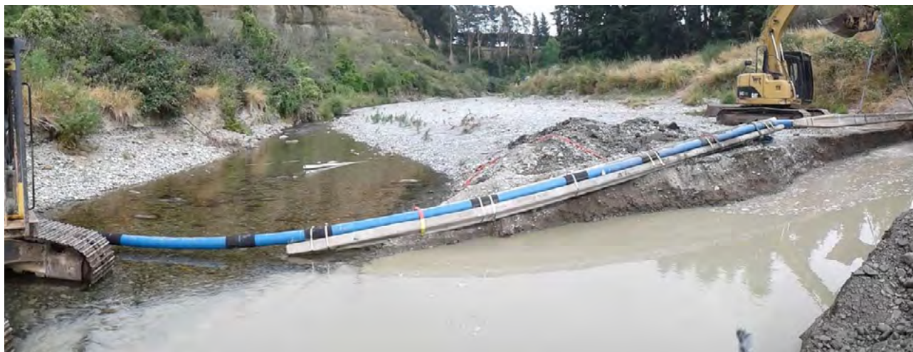
Iplex Poliplex® PE 100 pipe, installed in a river crossing, for a drinking water transmission main, Waitaki District.
