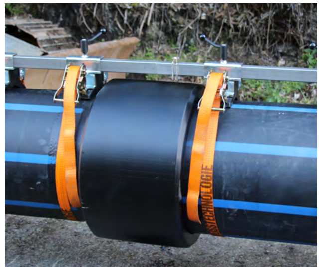
Iplex Poliplex® PE 100 pressure pipe showing electro fusion welding.
