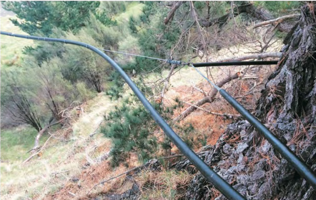
Iplex Blackline™ HP PE 100 pipe, installed in an aerial river valley crossing for stock water supply, Pohangina Valley, Manawatu District.
