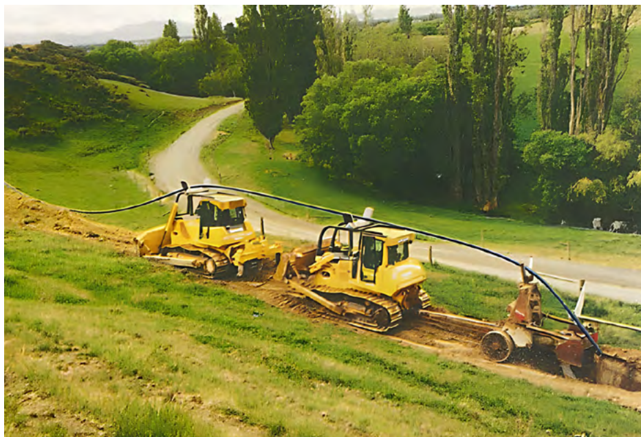
Iplex Blackline™ PE 100 pipe installation by mole ploughing, for stock drinking water supply.
