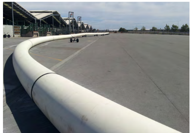
Iplex Poliplex® DN710, PN12.5, PE 100 sewer rising main being prepared for installation by horizontal directional drilling, in Christchurch City. Pipe is black with a cream coloured jacket, identifying it visually as a pressure sewer in accordance with AS/NZS 4130.
