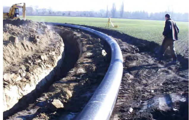
Curved Poliplex® PE 100 pressure sewer transmission main, Timaru District.
