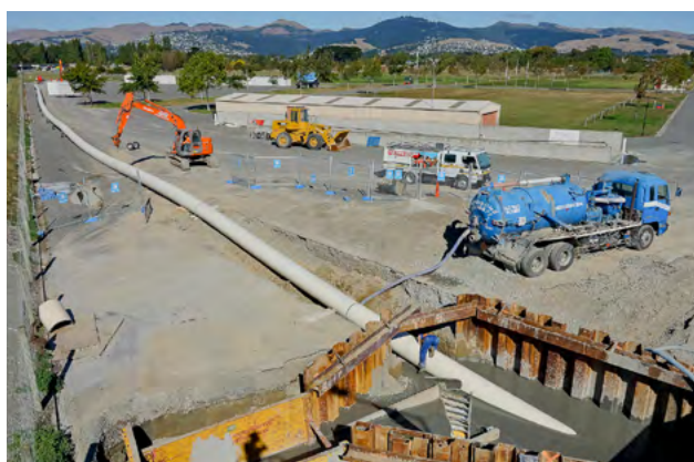
Iplex Poliplex® PE 100 pressure sewer transmission main, installed by Horizontal Directional Drilling, Christchurch City.
