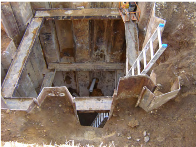
Figure 2.1 Restrain® installation by Auger Boring, at 10.8 metres to invert
