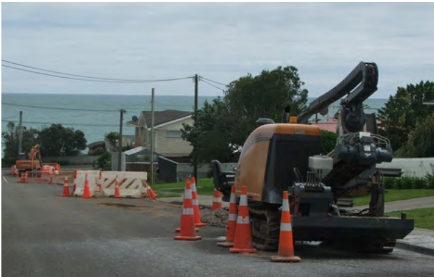
Figure 7.1 Typical cartridge style HDD pull-back.
