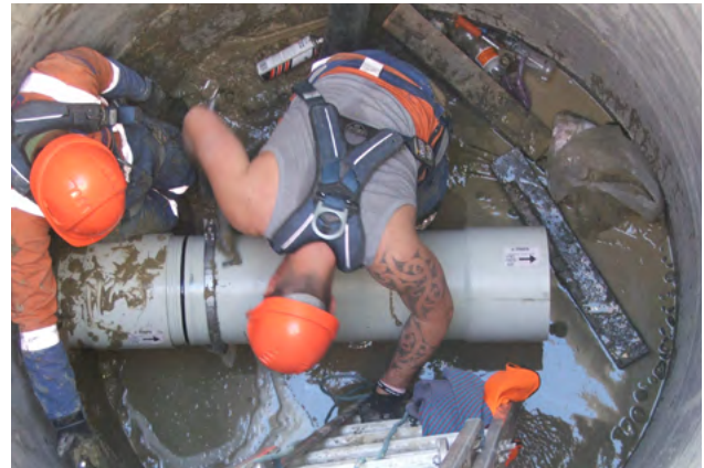
Figure 7.2 Typical HDD cartridge style pull-back within a 1.8m diameter x 4.5m deep manhole structure installing DN300 x 1m Restrain® Sewer Pipe.
