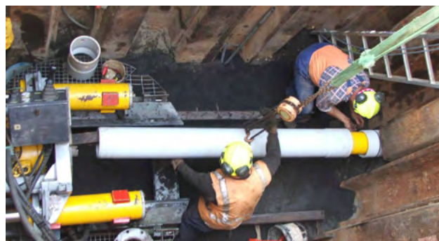
Figure 7.16 Typical Micro Tunnelling installation.
