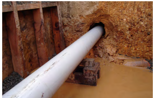
Figure 4.3 Restrain installation by Pipe Reaming of an earthenware host
