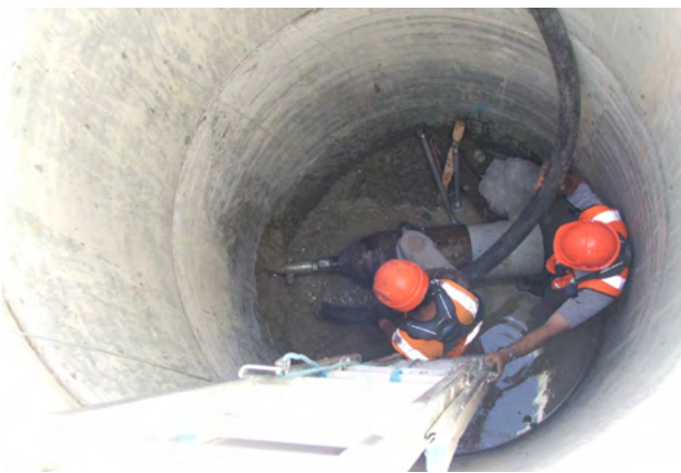
Figure 4.1 Restrain installation by Horizontal Directional Drilling
