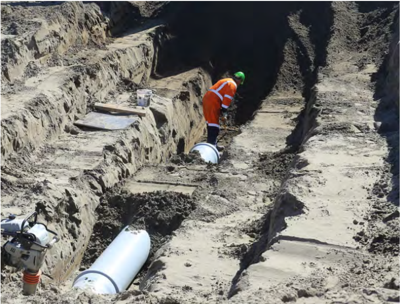
Construction of Iplex Superstorm® PVC-U stormwater drains. Mackays to Pekapeka expressway, Kapiti Coast.
