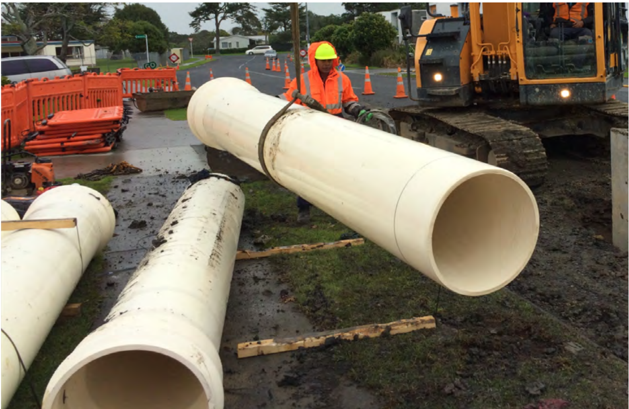
Installation of DN 600 Iplex Novadrain® PVC-U pipe for a transmission sewer pipeline in Mangere, Auckland City.
