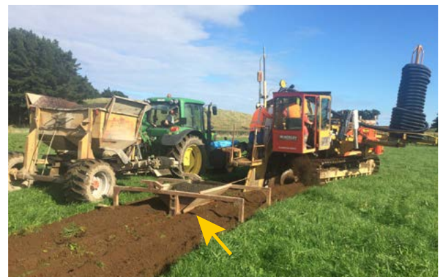
Introducing filter aggregate backfill as the NEXUSFLO™ pipe is laid
