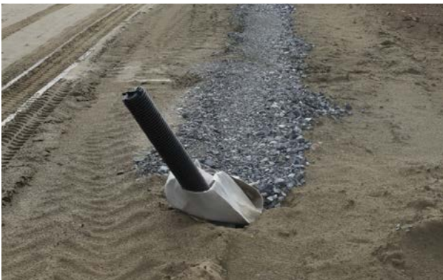
Access point in a NEXUSFLO™ drain system for water jetting
