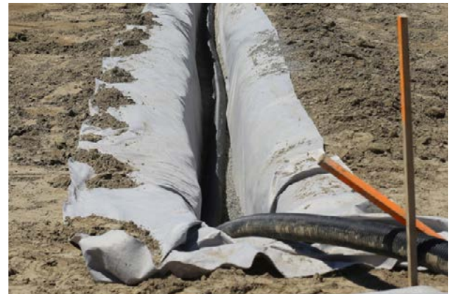
NEXUSFLO™ installed with geotextile surround of the drainage aggregate bedding and backfill envelope, in mobile sandy soil
