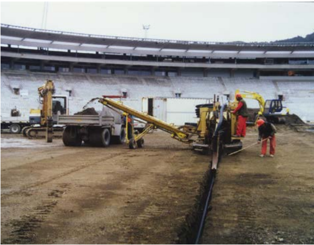
Wellington Sports Stadium. Installing Iplex NEXUSFLO™ during construction.
