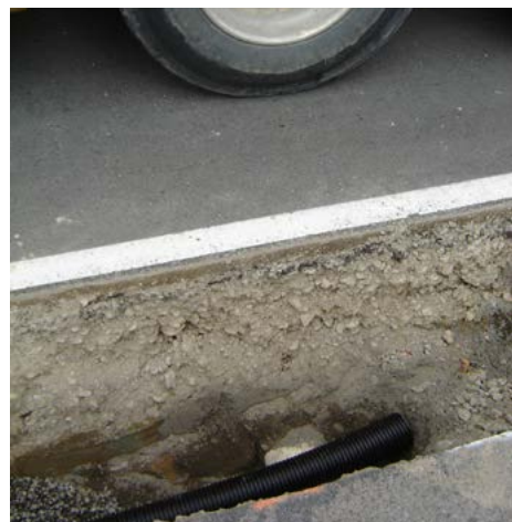
NEXUSFLO™ under a sealed commercial road, surrounded by permeable aggregate backfill, thoroughly compacted to NZTA Standard
