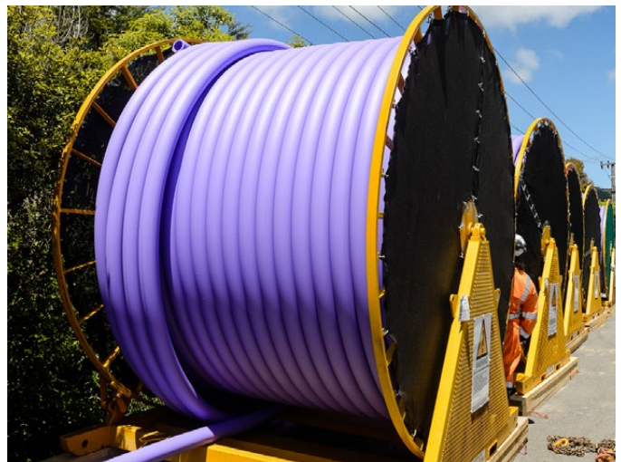
Drum Coils – DN 110 PE Communications duct SDR17
