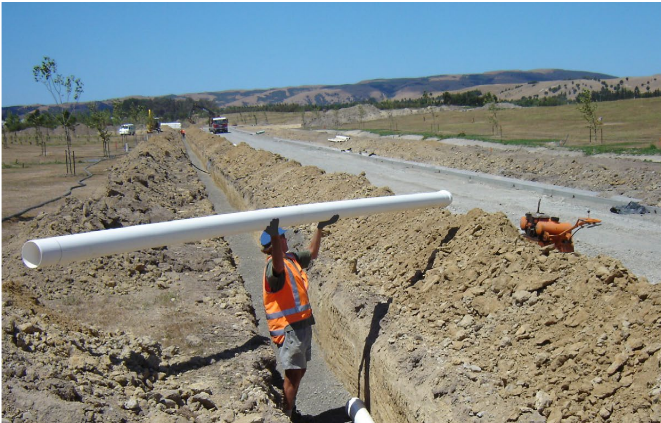
Image 1. Iplex PVC-O Pressure Pipe being installed
