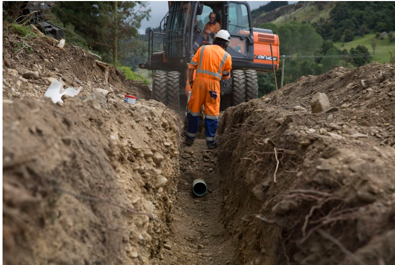
Photograph 6: Compaction of embedment zone above pipe (Image courtesy – Iplex Pipelines NZ Limited)
