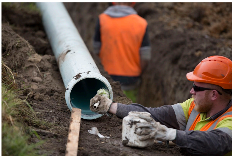
Photograph 5: Application of bactericidal pipe jointing lubricant to the locked-in-place seal ring (Image courtesy – Iplex Pipelines NZ Limited)
