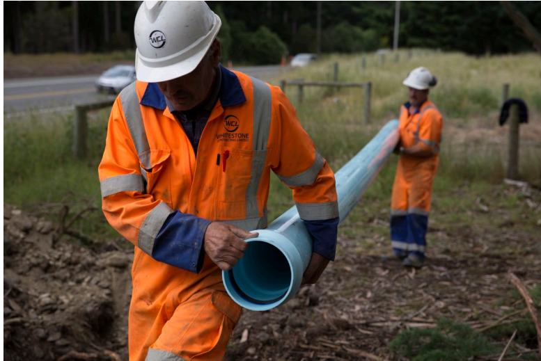
Photograph 4: Site handling a 6.5 m length of DN200 Series 2 PVC-O (Image courtesy – Iplex Pipelines NZ Limited)
