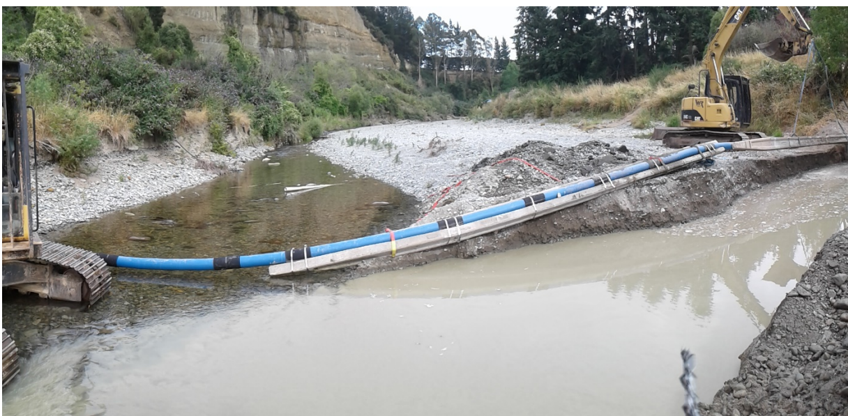
Photograph 7: Waianakarua River Crossing utilising concrete poles for anchorage. (Image courtesy – Waitaki District Council & Whitestone Contracting)
