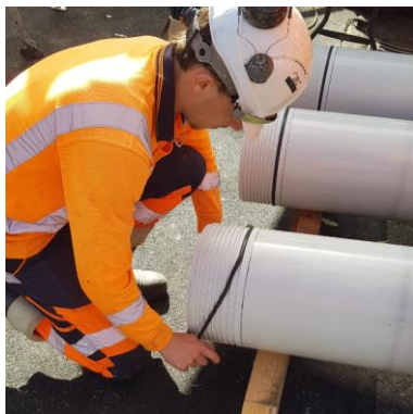
Fitting the Seal Ring
