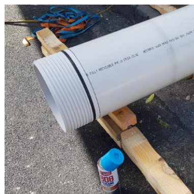
Approved Silicon Spray Lubricant Applied
