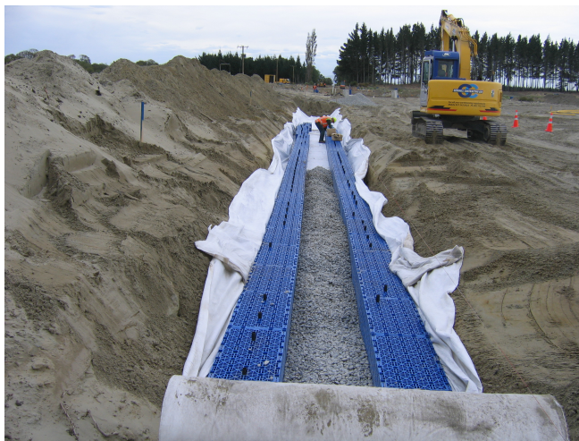
Wrapping an Aquacell™ infiltration gallery in geotextile fabric prior to backfilling.
