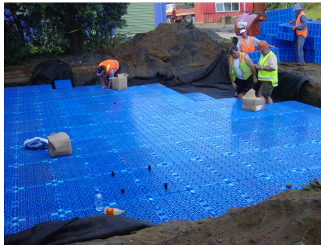
Aquacell™ attenuation and infiltration gallery under construction.
