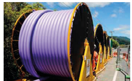
Drum Coils - PE telecommunication duct SDR17
