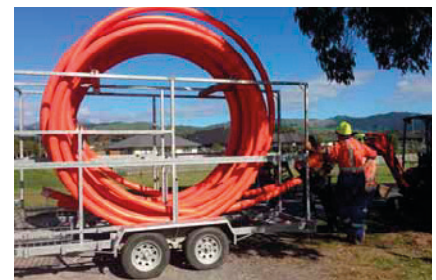
Two DN 110 PE electrical ducts in 50m coils on a dual-coil dispensing trailer.
