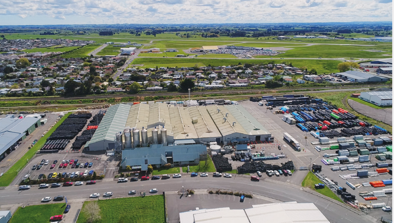
Iplex Pipelines manufacturing plant and distribution hub in Palmerston North city, New Zealand.
