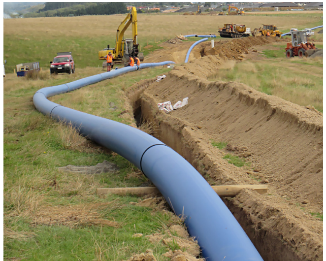
POLIplex DN 500 PN PE100 pressure pipe coloured black with blue jacket identifying it as a pressure water mains, Manawatu.
