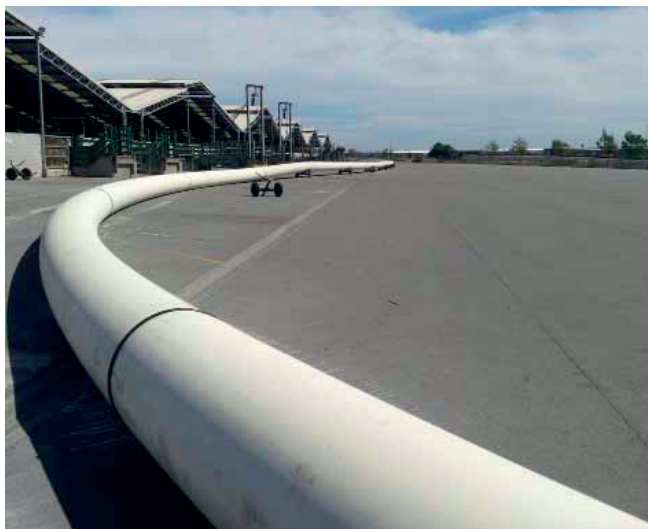
DN710, PN12.5, PE100 sewer rising main being prepared for installation by horizontal directional drilling. Pipe is black with a cream coloured jacket, identifying it visually as a pressure sewer in accordance with AS/NZS 4130, Christchurch City.
