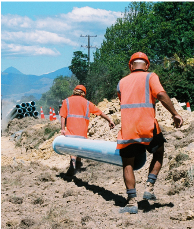
Site handling of light weight DN 250 S2 PN 16 Apollo in 6m lengths, near Nelson.
