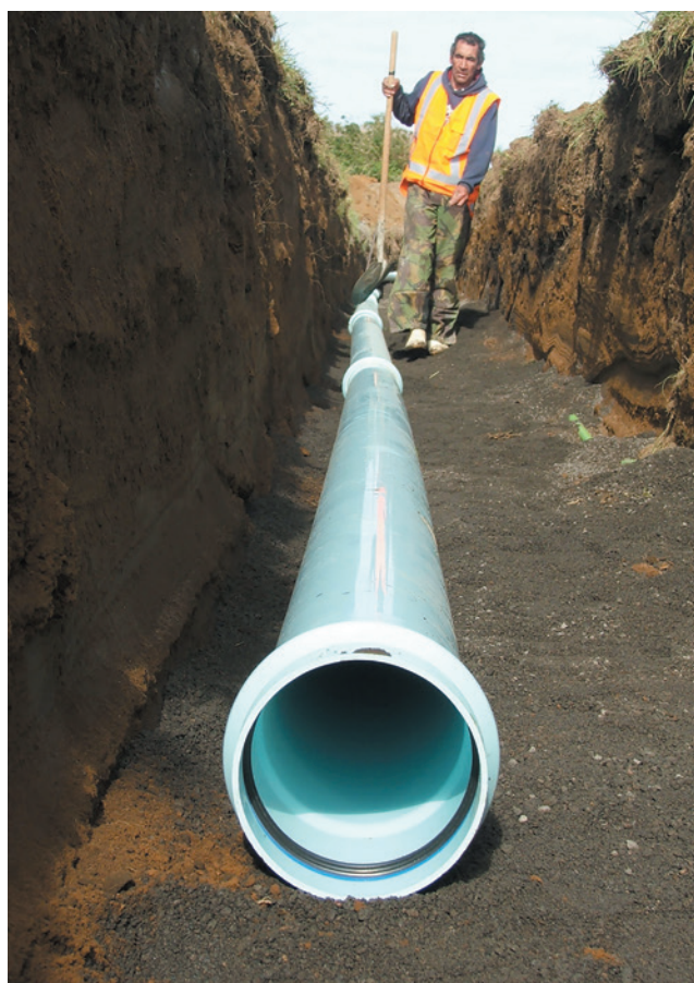
Installing a DN 150 S2 Apollo PVC-O Sewer Rising Main near Oakura, Taranaki.
