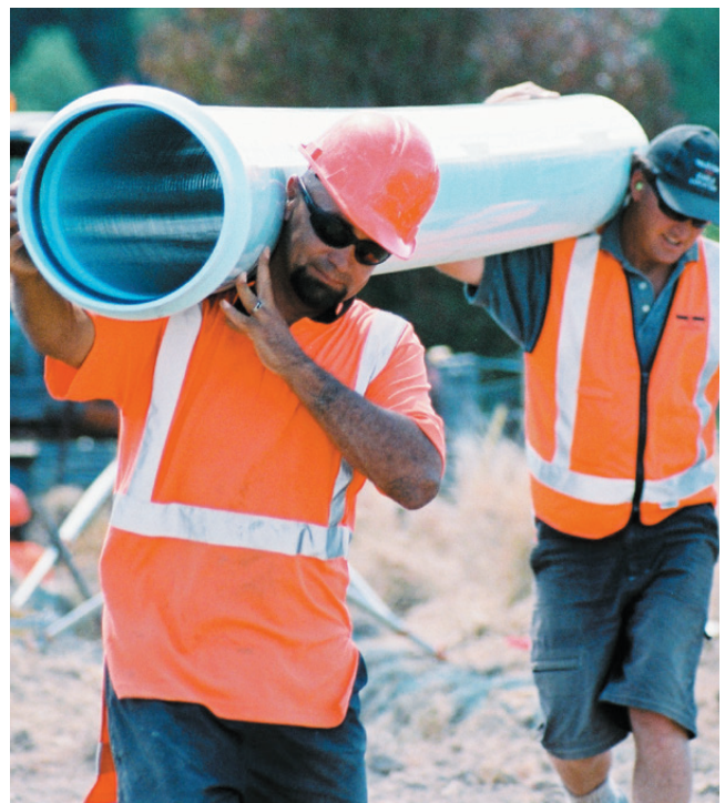
Easy site handling of light weight DN 250 Series 2 PN 16 Apollo Blue PVC-O pipe, with factory fitted, locked in place Blueseal rings.
