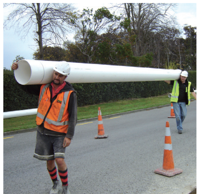
Site handling of light weight Apollo DN300 S1 PN12.5 in 6m lengths, Timaru city.
