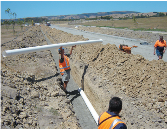
Site handling and installation of light weight DN 100 Series 1 PN 12.5 Apollo, for water distribution in a Residential Subdivision near Martinborough.
