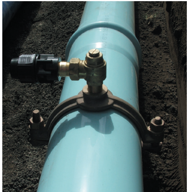
Installing a Milnes gunmetal tapping saddle and UPT ferrule with a Plasson lateral adapter, on DN 150 S2 PN 12.5 Apollo PVC-O pipe.
