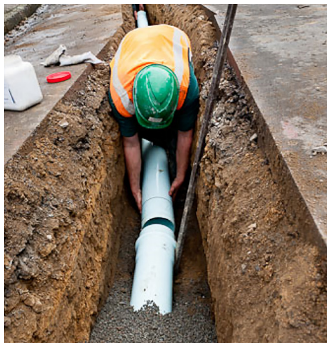
Assembling a joint on DN 150 S2 PN 16 Apollo PVC-O in Wellington City.
