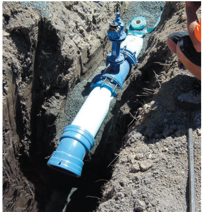
Ductile iron socketed bend and AVK flange adapters being installed on a DN 250 S2 PN 16 Apollo PVC-O watermain near Nelson.
