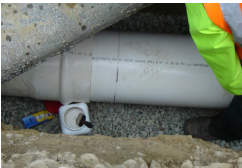
Figure 6.17 - Insert aligned lubricated spigot into socket
