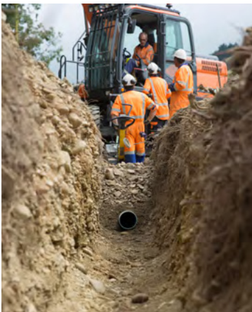
Figure 6.25 - Showing correct position of pipe, fully surrounded by selected size imported bedding aggregate, with all other larger size "as dug" aggregate, totally excluded from direct contact with the pipe, Waitaki District
