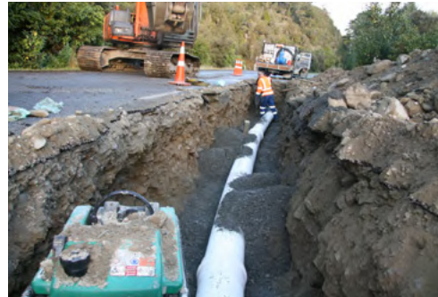
Figure 6.26 - DN300 Iplex PVC Series watermain, in 6m lengths, following a curved road alignment, Westland District
