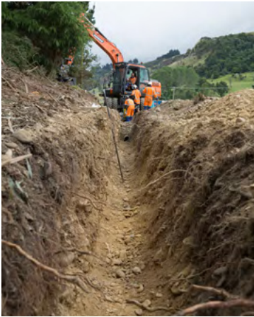
Figure 6.23 - Trench bottom in stoney ground, evenly cut to grade and depth before placing the bedding aggregate. Waitaki District
