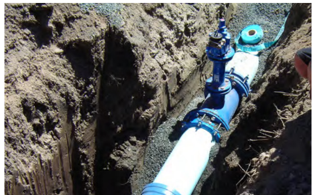
Figure 3.11 - Typical arrangement of "AVK" brand, Universal flange adapters, on a flange branched tee, with hydrant, and hydrant riser, installed onto Iplex® PVC pressure pipe, Tasman District
