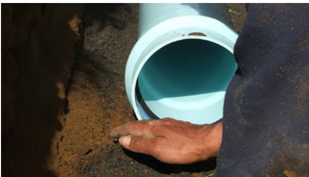
Figure 6.10 - Carefully clear away any dirt from the socket mouth
