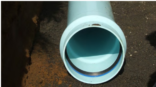
Figure 6.11 - Totally clean socket, ready for jointing
