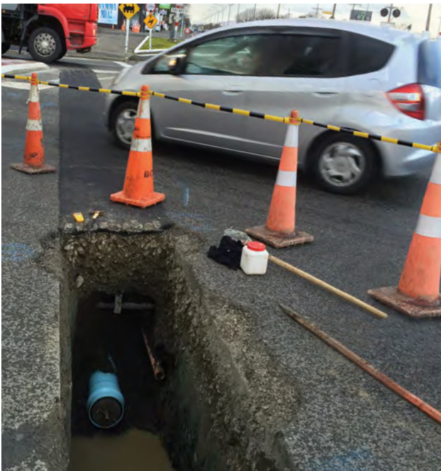
Figure 5.1 - Iplex PVC DN150 S2 pressure watermain installed under SH 54, Feilding Town Centre, Manawatu District
