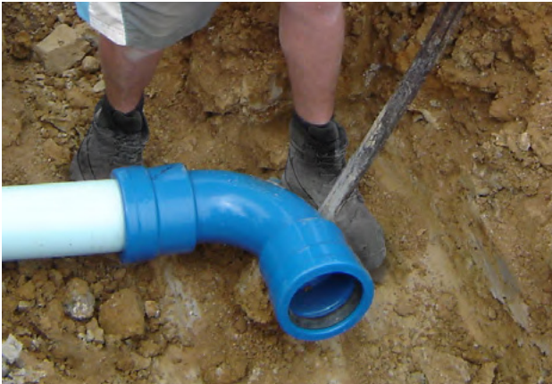
Figure 3.6 - Assemble the fitting onto the PVC pipe with a bar. Insert the pipe into the full length of the fitting socket
