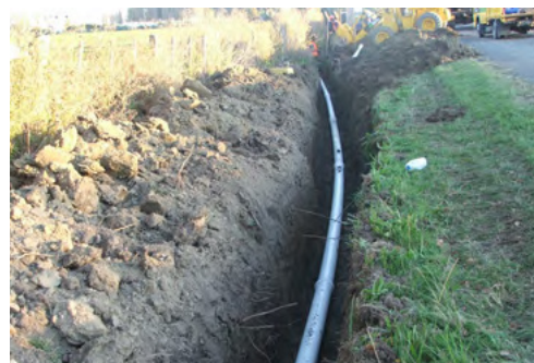
Figure 6.29 - DN100 Iplex PVC waste water transmission main, in 6m lengths, on a curved alignment, Gisborne District
