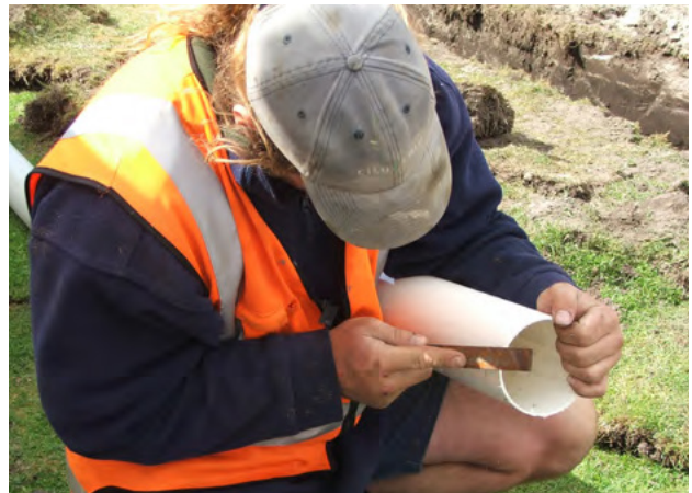
Figure 6.8 - Chamfering pipe with hand file
