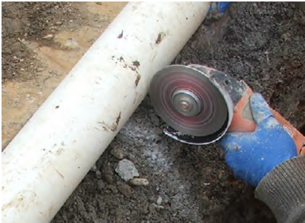
Figure 6.5 - Cutting pipe with power-driven masonry blade
