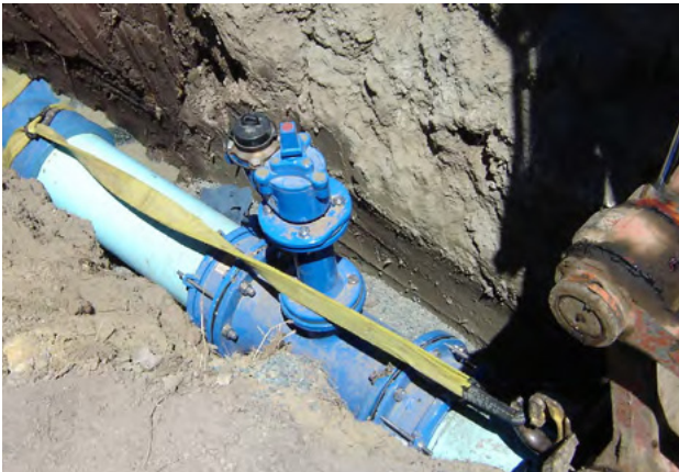
Figure 3.7 - Larger size ductile iron fittings may need extra mechanical help to assemble, such as here, with a lifting strop pulled by the excavator. DN250 socketed bend being assembled onto a DN250 Series 2 Iplex® PVC watermain near Richmond, Tasman District
