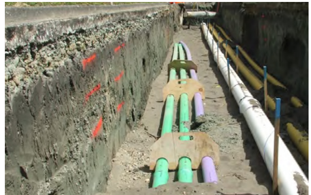
Figure 5.2 - Trench with temporary red index marks on the trench wall to guide backfilling and compaction in 300mm layers
