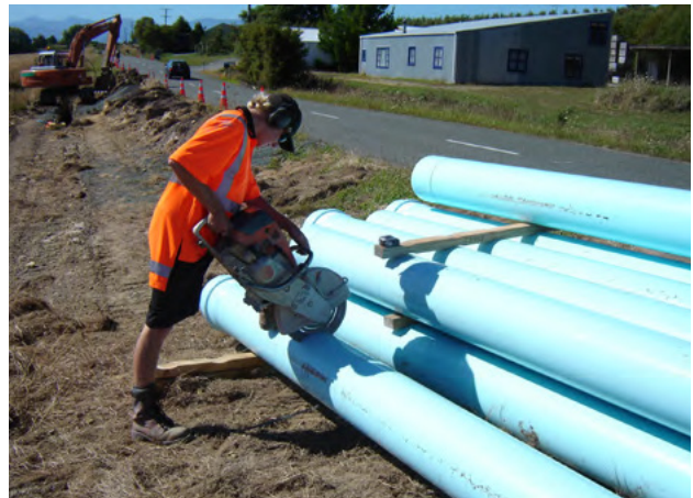
Figure 6.7 - Cutting pipe with power-driven masonry blade
