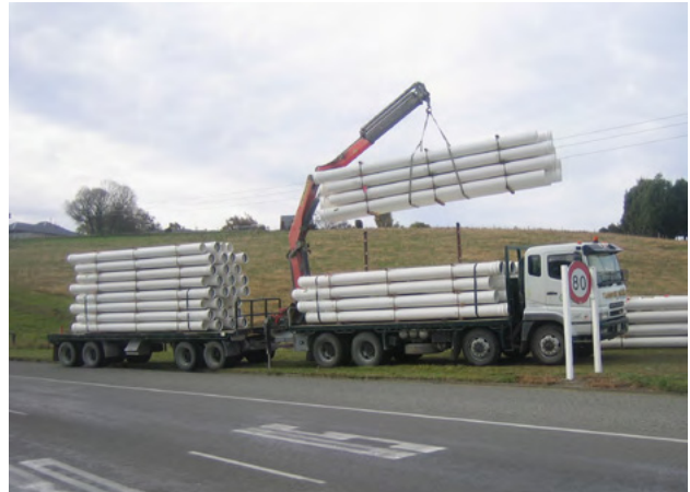
Figure 6.2 - Mechanical lifting, using two point suspension, and polymer slings, of DN300 Series 1 Iplex PVC pipe in bulk crates, Timaru City
