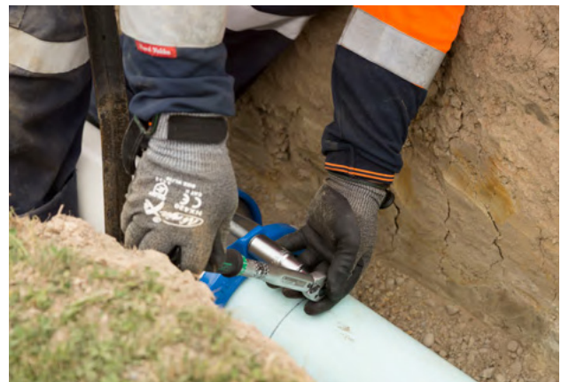
Figure 3.10 - Use of a torque wrench during final tightening of the bolts on an "AVK" brand Universal Coupling, installed on DN100 Series 1 Iplex® PVC pressure pipe
