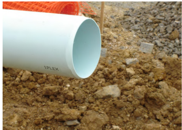
Figure 6.9 - Hand- chamfered Iplex PVC pipe spigot
