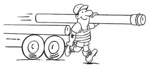
They're so light these days; I can unload a truck quickly – one at a time – **NEVER TIP THEM OFF!** Then I have to store them correctly on dunnage, on flat ground with supports. Iplex pipes have scalloped timber dunnage these days, so when I cut the pipe packs open they don't roll everywhere!
