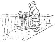
If I do the compaction correctly I never need to be called back to the job to correct slumped trenches. I never get paid for doing a job twice... any call backs are on me!
