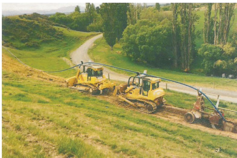
Mole Plough installation of Iplex Blackline pipes.
