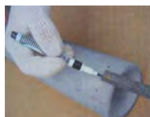
1. Marking: Use a pen and tape measure to place marks 25mm from the end of each pipe.
