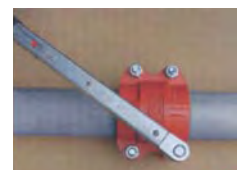
4. Tightening Nuts: Using an appropriate tool, tighten the nuts sequentially until the fittings' housing bolt pads meet, metal to metal.
