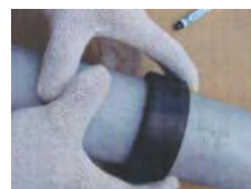
2. Gasket Mounting: Using a silicone based lubricant; slip the gasket over the pipe ends and center the gasket between the marks. Ensure the pipe ends are butted together.
