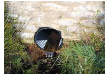
Cost effective culvert
